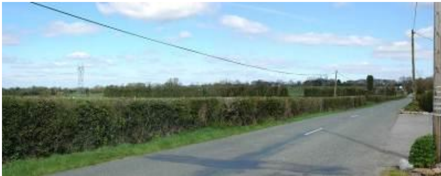
View 76 from the R125 at Leonardstown showing existing (single circuit) 400 kV electricity line
